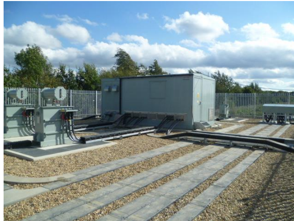
Figure 5 – Substation Upgrade works at Gatwick
