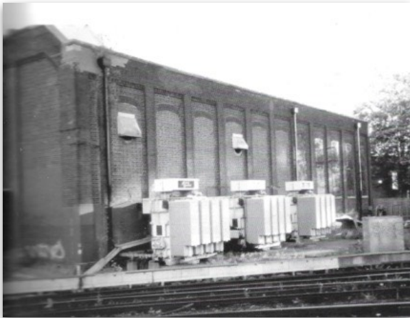
A twenty-first century view of Waterloo substation. Note the 'new' transformers outside, these would have been at least the third set installed since the substation was built for the original LSWR electrification. (Peter Winchester)
