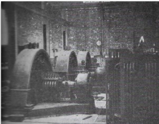
Interior of Waterloo substation. On the left of this view is the direct current switchboard and, in the centre, three of the rotary converters. At the right hand ends of the converter shafts can be seen the the small synchronous motors used to start the machines, and in the centre there are the six slip rings. Just visible is one of the substations transformers. (Railway Magazine Archive)
