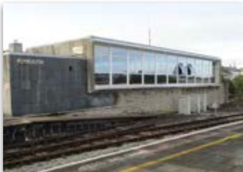
1960s Power Box
