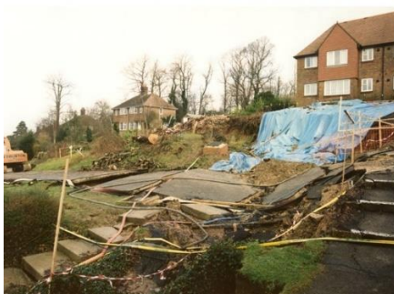
FRANKLANDS VILLAGE LANDSLIP
